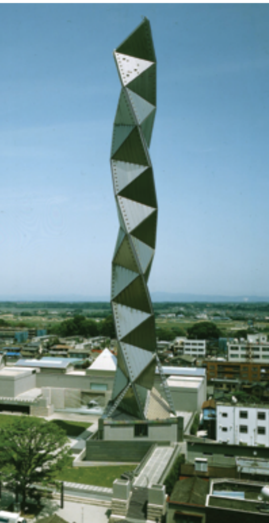
This tetrahelix structure was designed by Arata Isozaki and built in 1990 in Mito, Japan. (Photograph courtesy of Art Tower Mito, Japan.)
